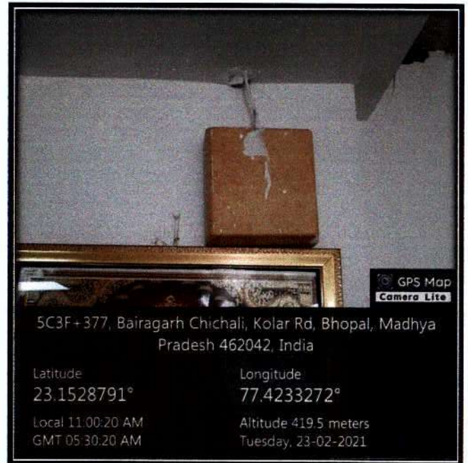
Booster Office- Ground Floor
