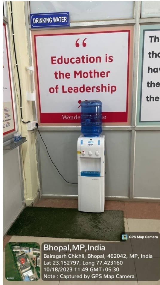
Drinking Water Facility
